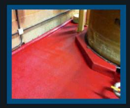
By using our vinyl ester linings we can repair spalled and eroded concrete and return the concrete to better than new construction. This allows the coating to handle the acids and caustics and not permeate the concrete and leach chemicals into the ground water. Saves money and better environmental results when using our secondary containment coatings.
