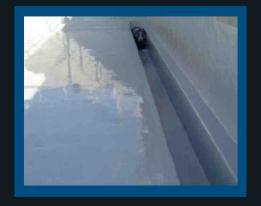
Chemical attack on concrete. Repaired with Milamar 2620 chemical resistant liner and topcoated with Milamar 3300 CR chemical resistant veilcoat.
