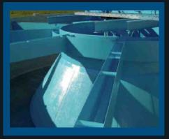
Blasted to near white metal and installed Chesterton ARC-S-1 PW potable water lining to all metal areas. Not only protected from erosion and corrosion the clarifier is easy to clean as the lime build-up is minimal. Less downtime saves money.
